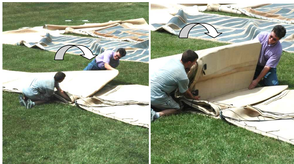
Figure 26 – “Accordion” fold the solar panel area of the fabric
