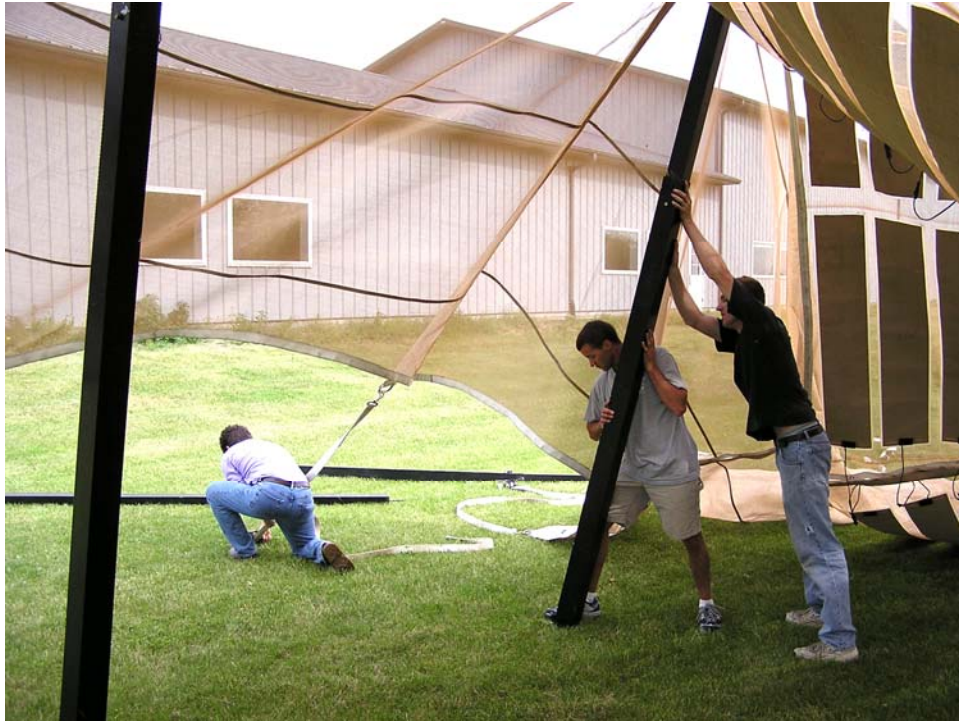
Figure 24 – Install First Pole
