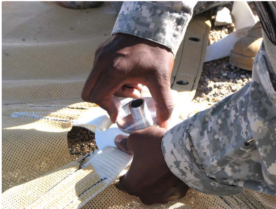
Figure 12 - Pole Plate Assembly
